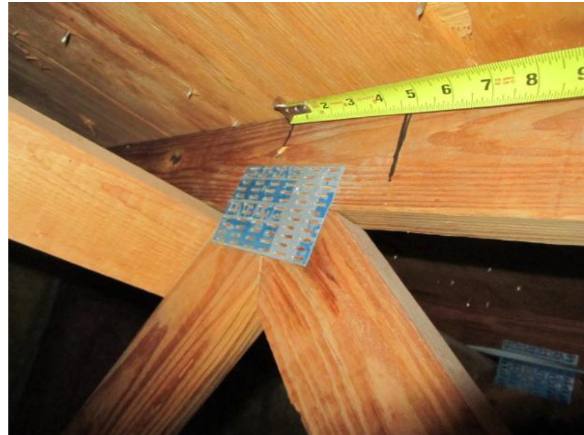
8d Nails Spaced 6" x 6"
