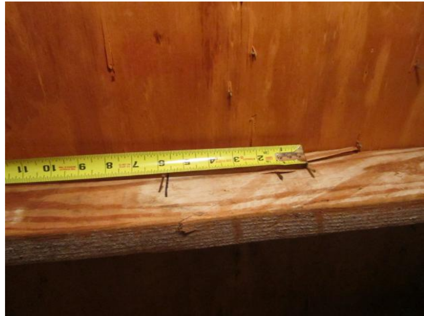
8d Nails Spaced 6" x 6"
