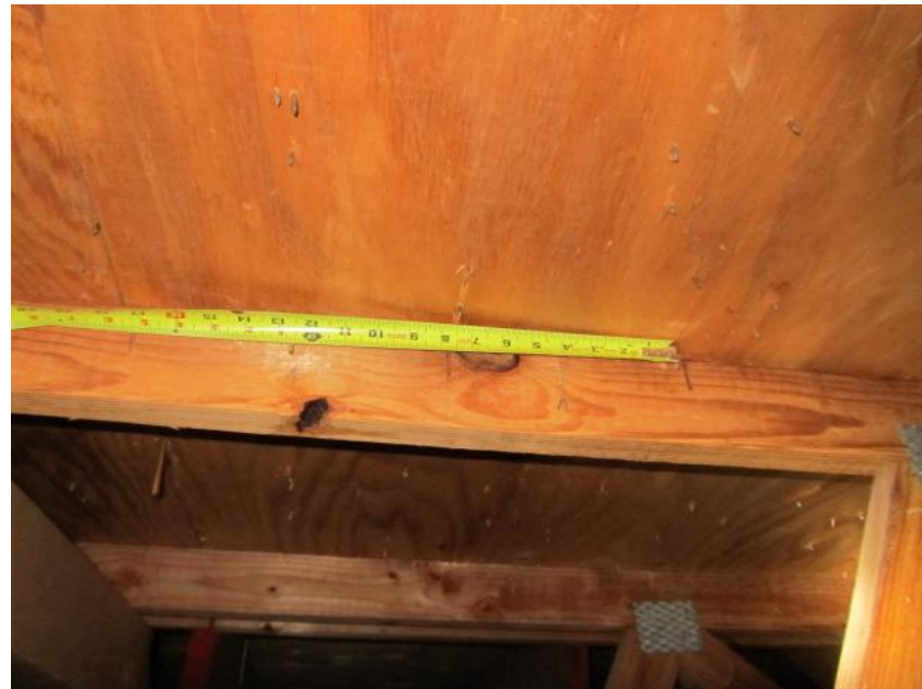
8d Nails Spaced 6" x 6"
