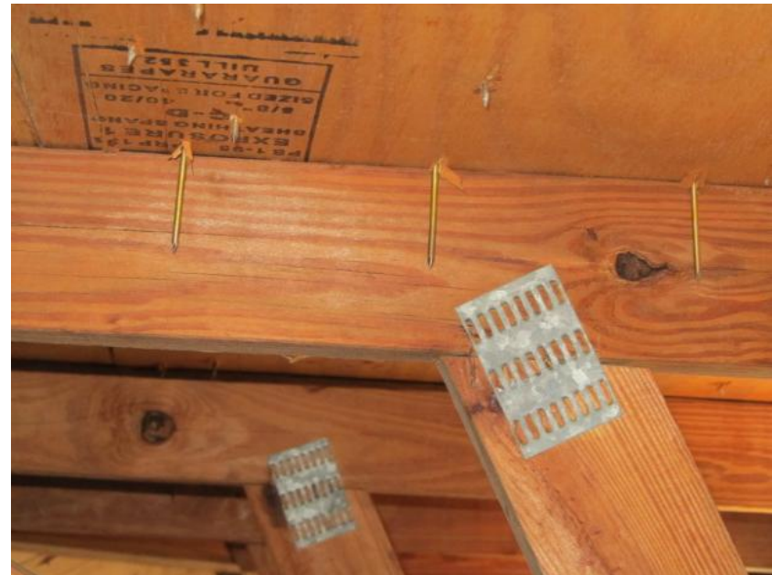
8d Nails Spaced 6" x 6"
